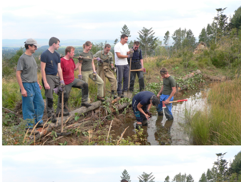
Fig. 35 A Water Forest in the High Tatras – building water conservation measures on territory destroyed by a natural disaster An example of the renewal of vegetation and hydrological stabilization of a territory through the conservation of water on land.
