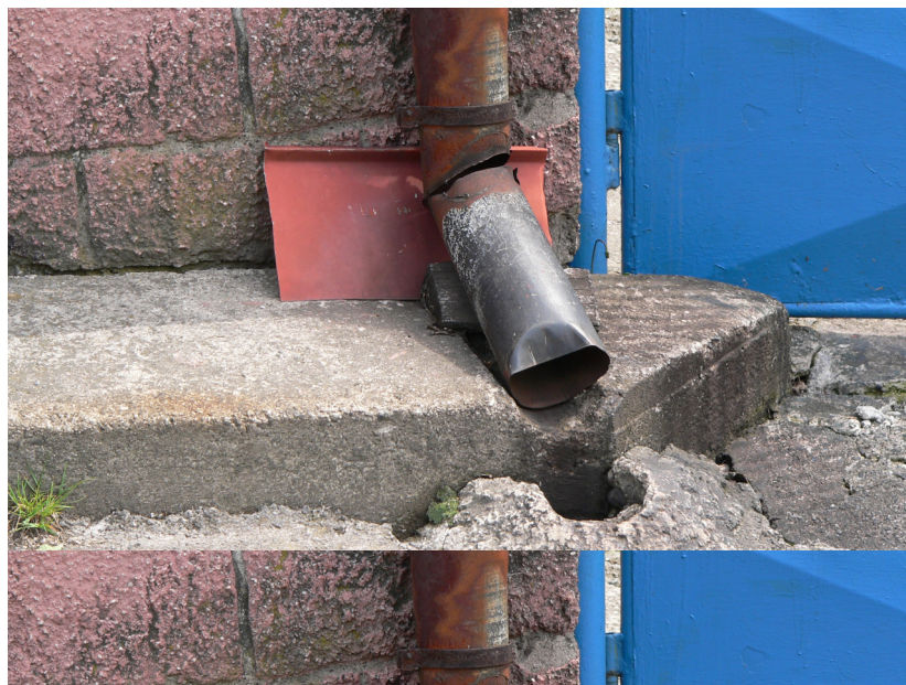
Fig. 13 The sluicing away rainwater
