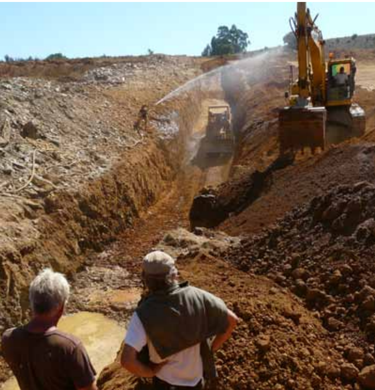
During the construction of a dam utilizing natural materials in 2011
